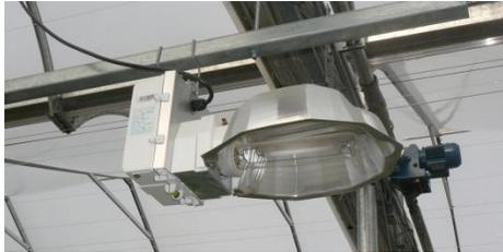
Figure 9. High Intensity Discharge (HID) luminaire in a greenhouse.
